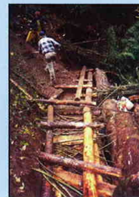
Before slope stabilization.
