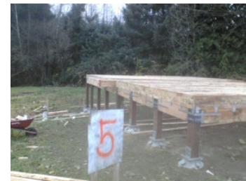
LID Foundation at Clearwater Commons in Bothell.
