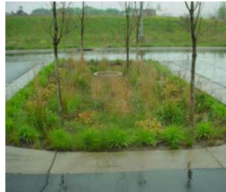
Areas proposed for infiltration need to be protected from compaction and sediment-laden runoff during construction
