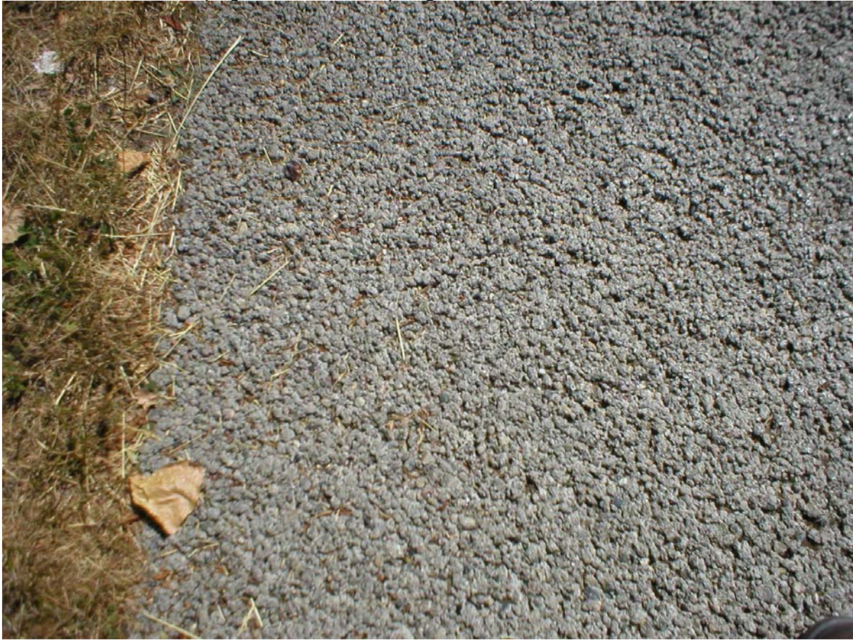
Photo 1. Sidewalk Sweeping- Left side un-swept, right side swept with Tenant Machine
