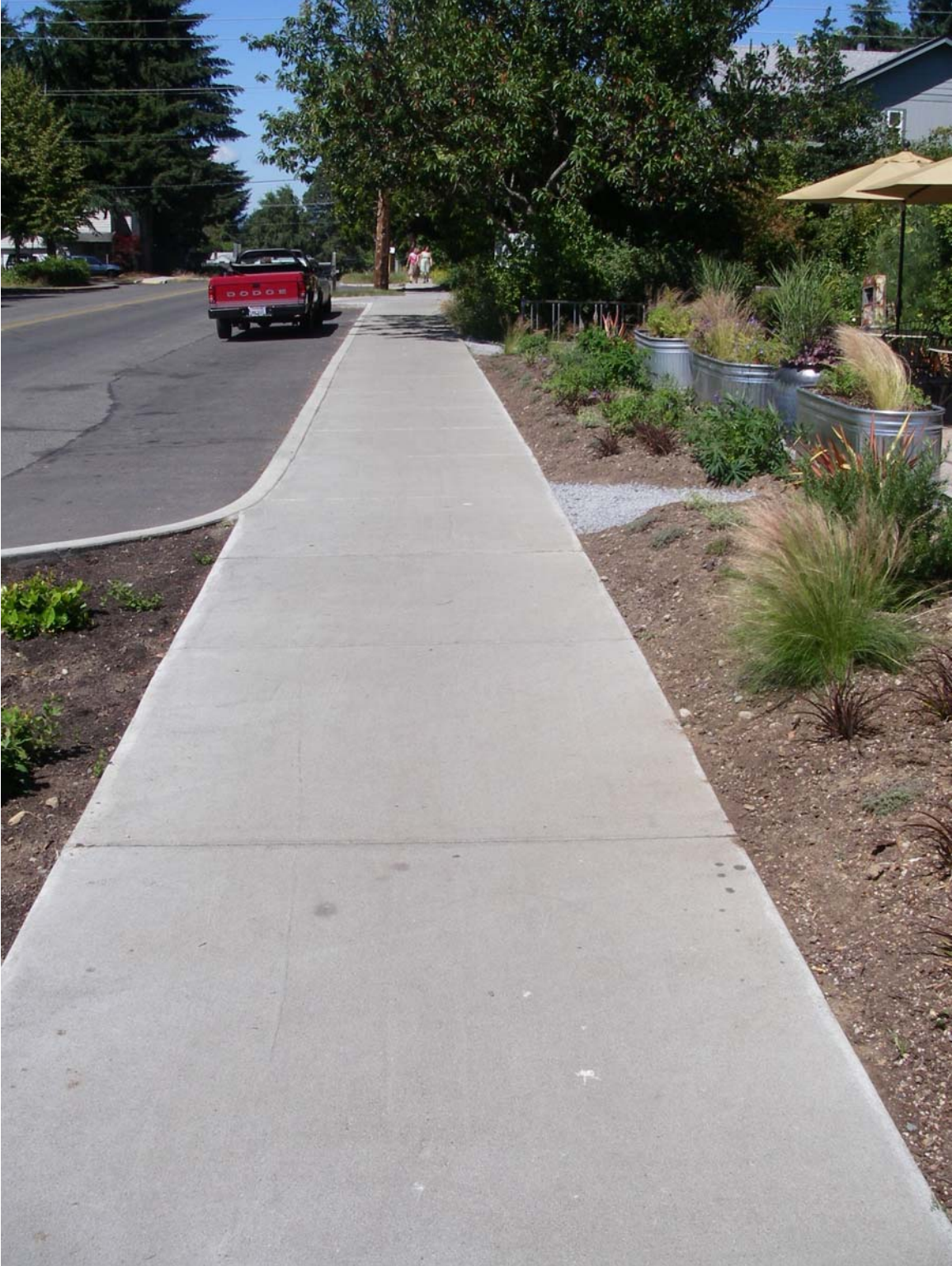
San Francisco Avenue porous concrete sidewalk adjacent to bakery.
