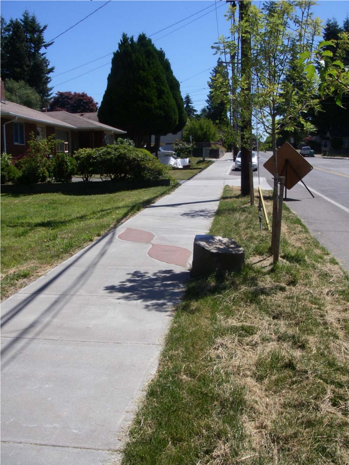
San Francisco Avenue porous concrete sidewalk showing art installation
