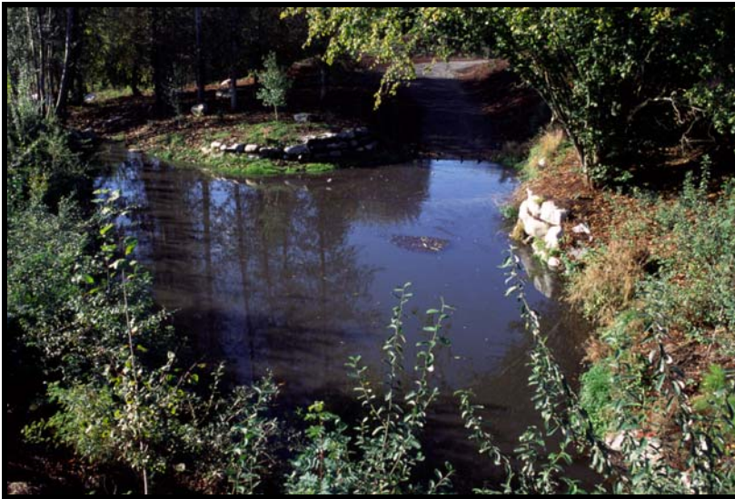
Indian Creek Stormwater Treatment Facility
