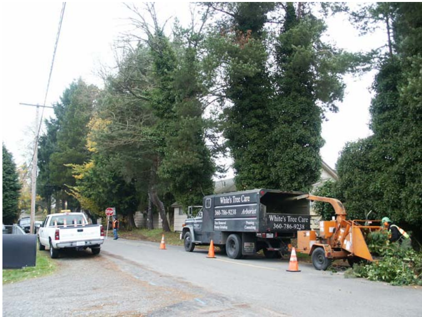
Devoe Street was one of the sites where hazard trees were removed and converted to firewood for low-income and underserved community members. Over 20 cords of firewood were collected from the removals.
