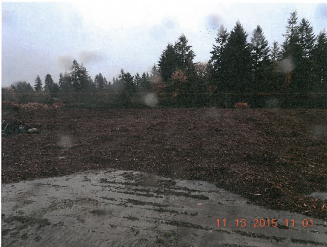
Concrete and brick were stockpiled to the left—verified as removed.
