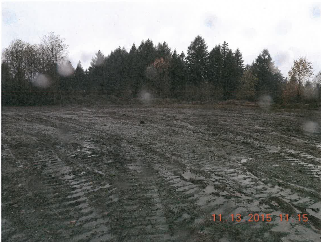
Area where imported soil piles were graded out.
