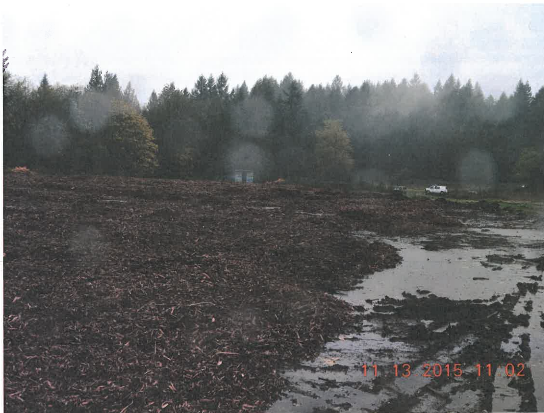
Chipped wood spread out, and providing erosion control for bare soil.
