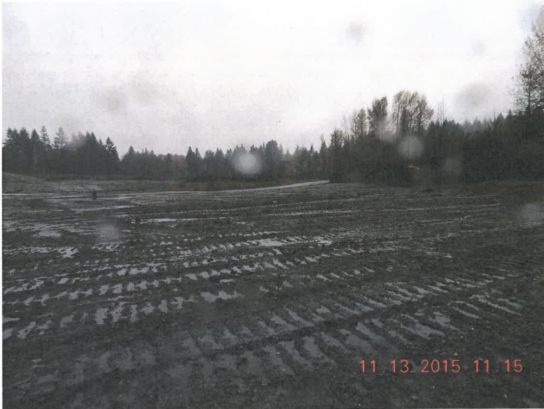
Another view of graded imported soils.
