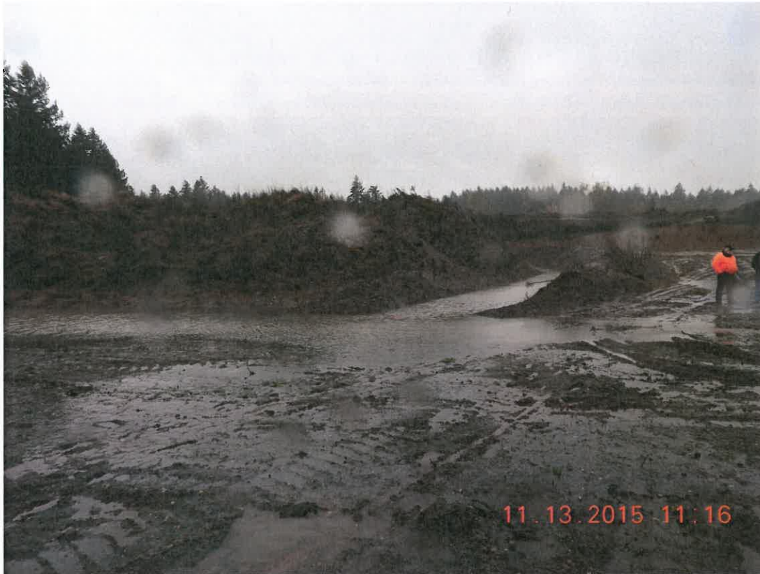
Looking NE—toward soils that were not disturbed by recent site activities.
