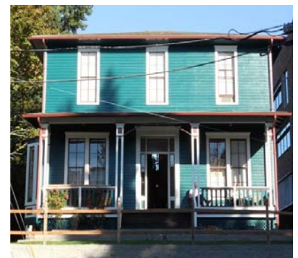
Steele House Apartments were built in 1869 and needed a lead-safe certified contractor to repaint the exterior, funded by CDBG. Funded by PY 2009 funds, completed in PY 2010
