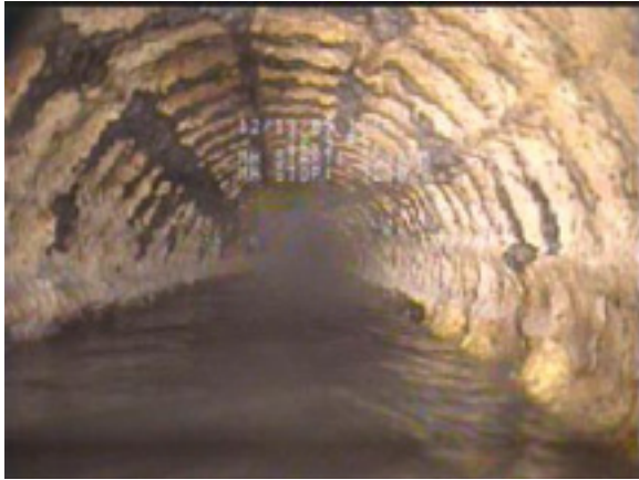
Sewer Line Televising/Inspection
