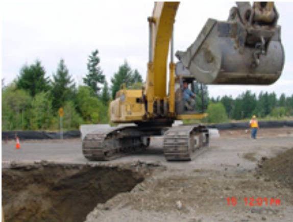
Sewer Line Construction
