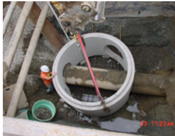
Sewer Line Construction
