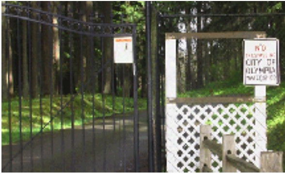
Water Supply Protection
