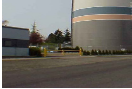
Water Supply Protection
