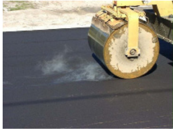
Asphalt Overlay
